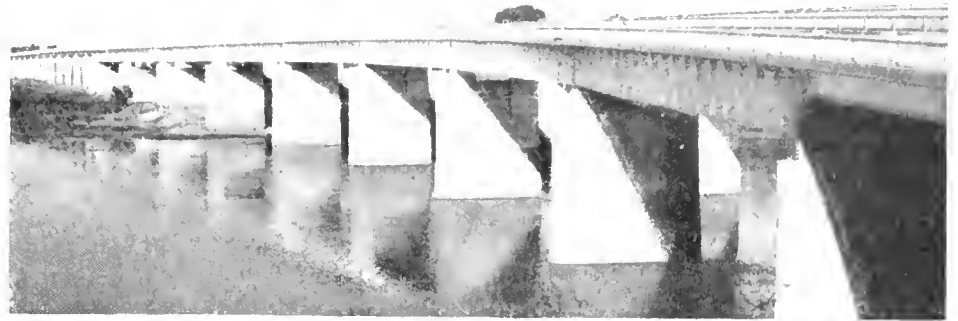
Two views (see also below) of completed Elvas Bridge which will be opened to traffic when the Elvas Freeway is completed
